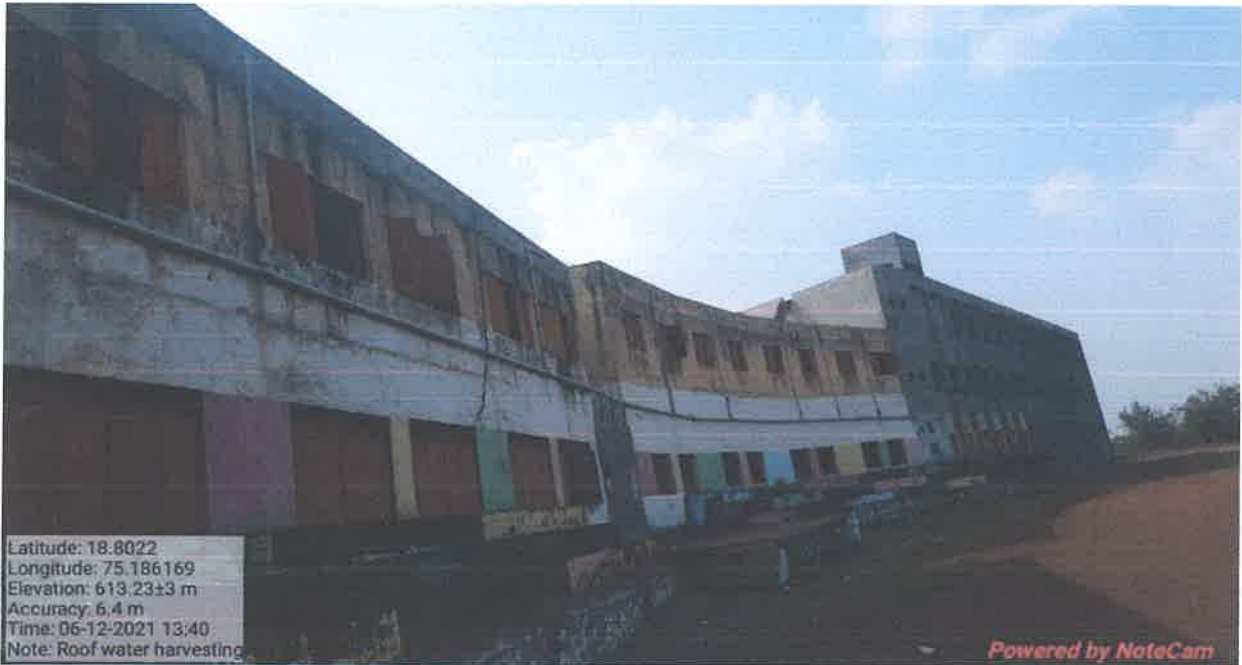
Rain Water Harvesting
