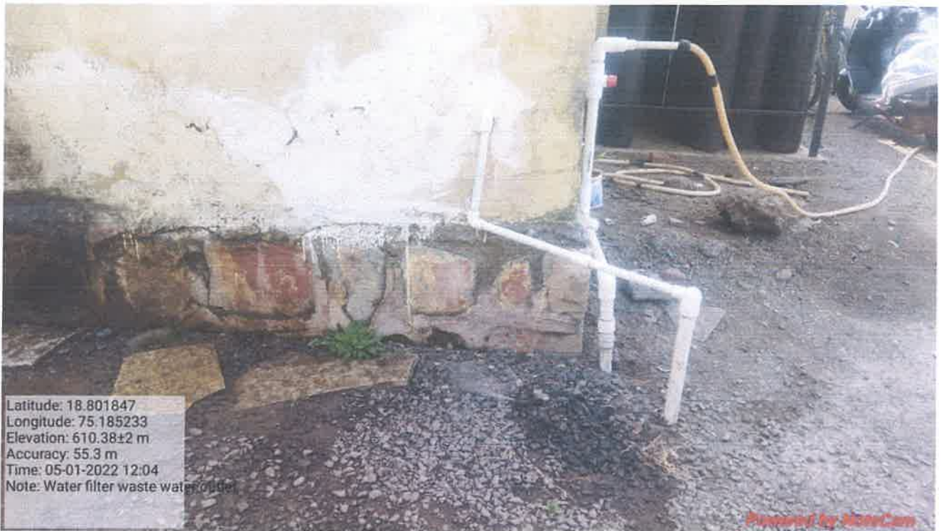
Water filter waste water outlet
