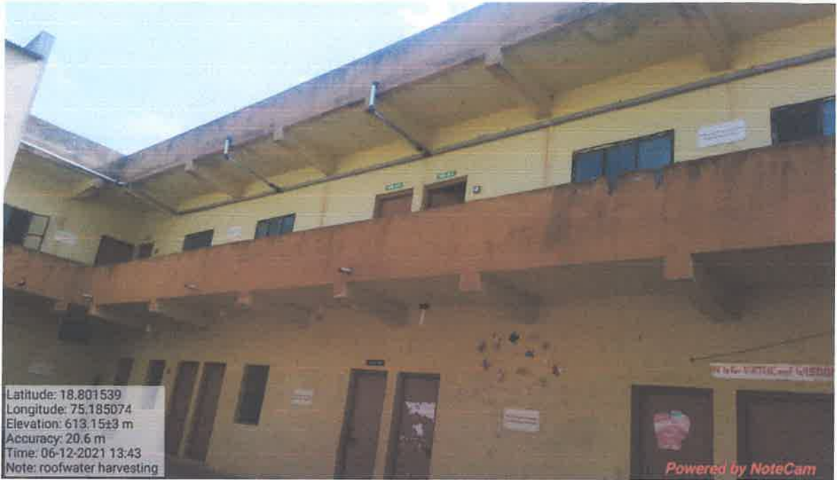
Rain Water Harvesting
