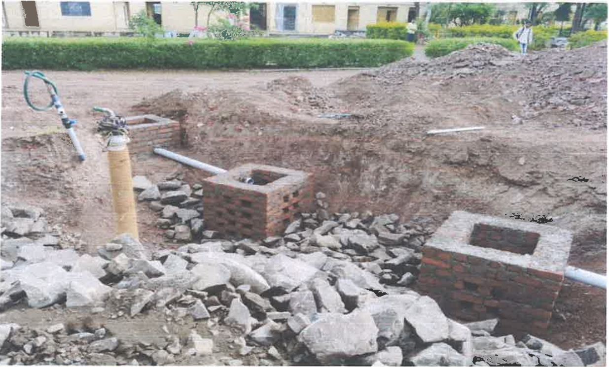
Bore-well Recharge system at the time of construction
