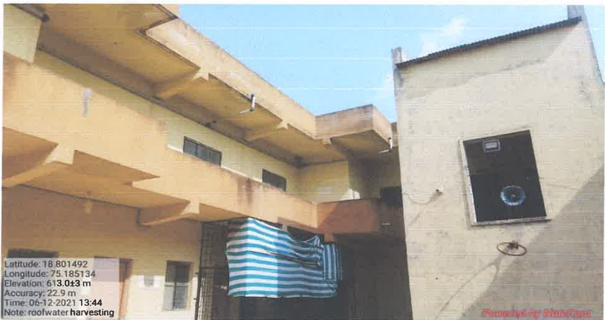
Rain Water Harvesting
